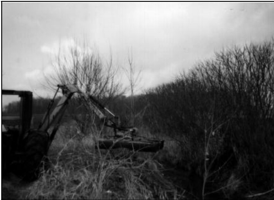
Exhibit 303a: Mechanized Debrushing Using Heavy Machinery (Source: Allen County Surveyor's Office Files)
