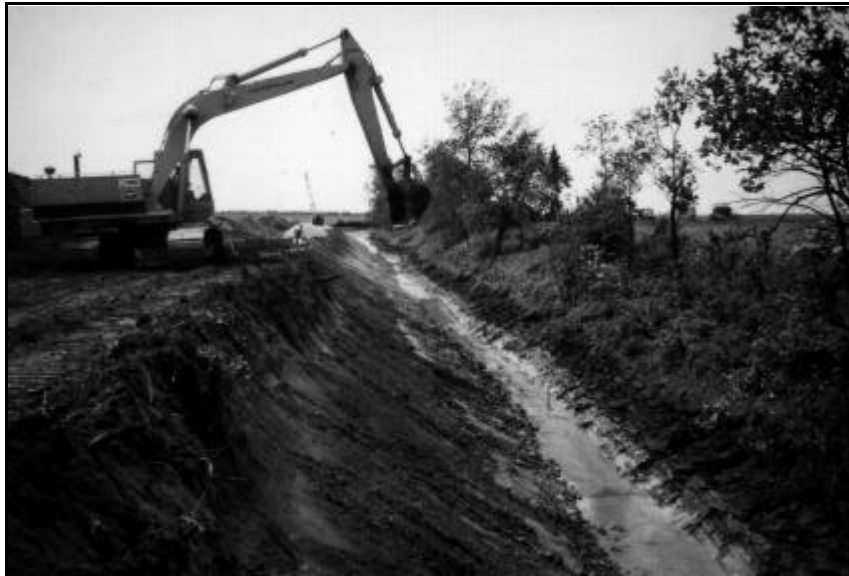
Exhibit 602a: Channel Excavation/Dredging (Source: NRCS Files)
